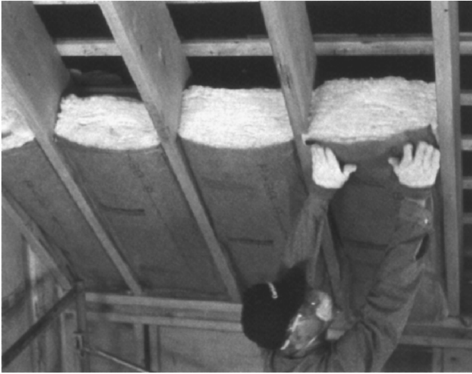
Figure 8.8 High-performance fiber glass batt. ( CertainTeed )
